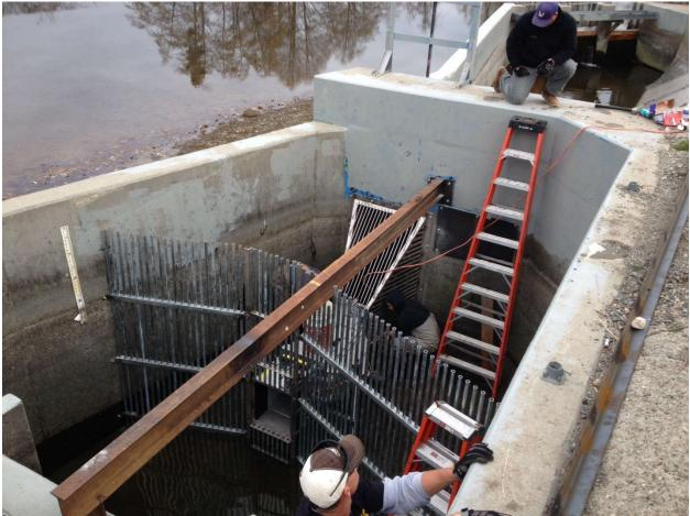
Figure 10. VAKI Riverwatcher installed in the fish ladder adjoining Durham Mutual Diversion Dam.
