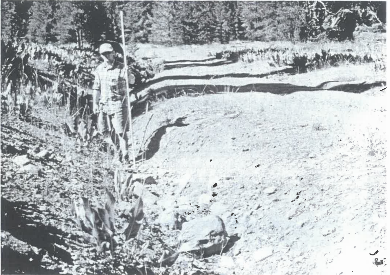
Many of the inboard ditches in the Scotts John Creek watershed are contributing fine sediments directly to streams.
