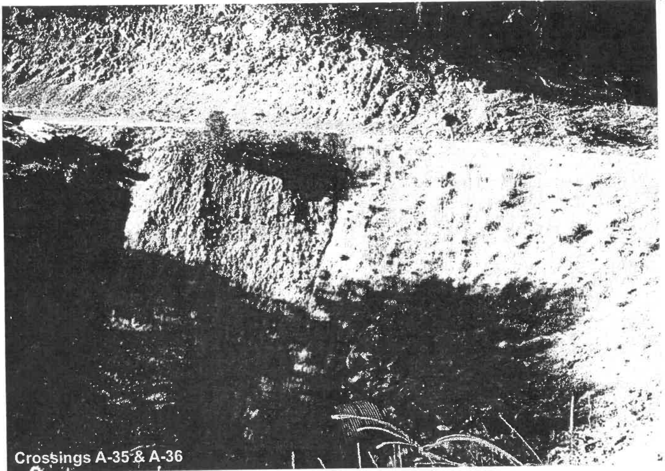
Two examples of fillslope erosion on the A-Line road in the Secret Creek Basin of the Bull Creek Watershed
