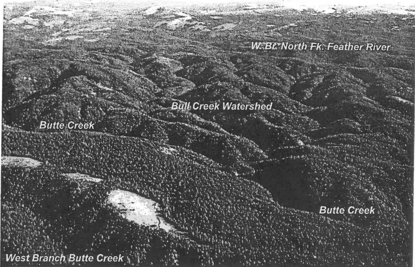
In the Bull Creek watershed (shown above), many of the stream crossing sites located on abandoned midslope roads have blown out, as in the example below.
